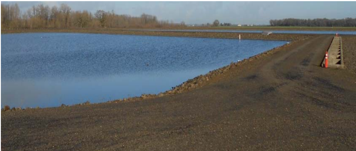
Wastewater Facility Lagoon 2
