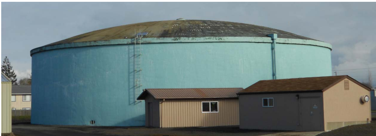
City's 2-Million Gallon Water Storage Tank
