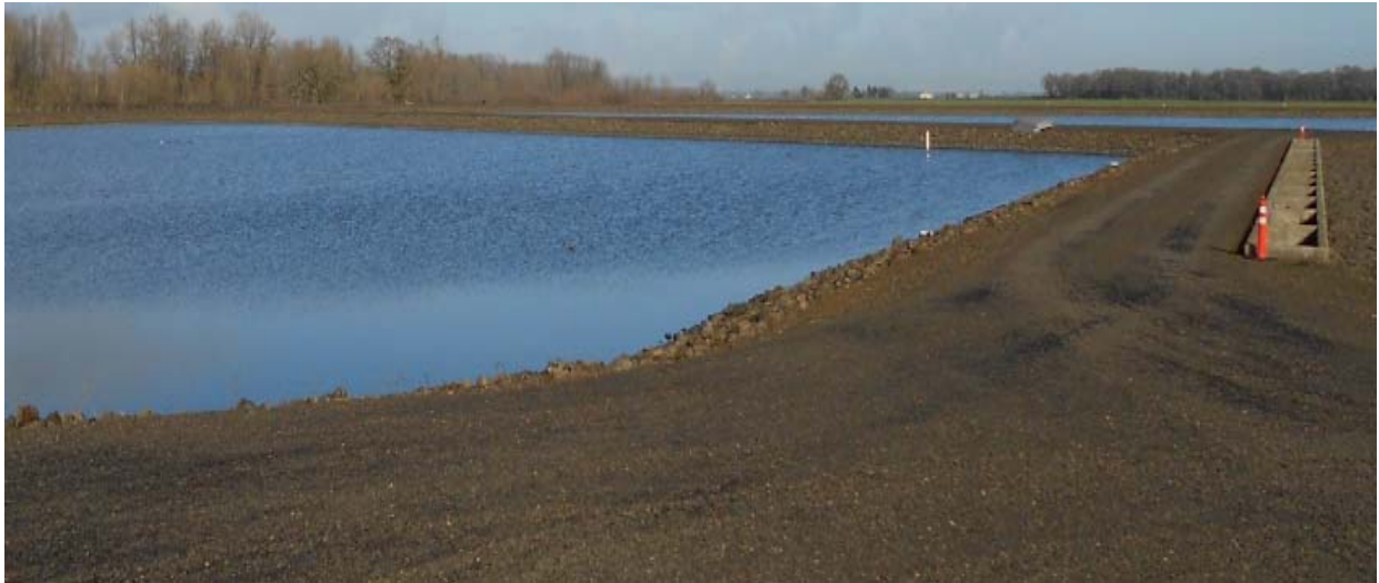
Wastewater Facility Lagoon 2
