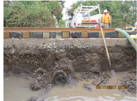
4th Street Railroad Project
