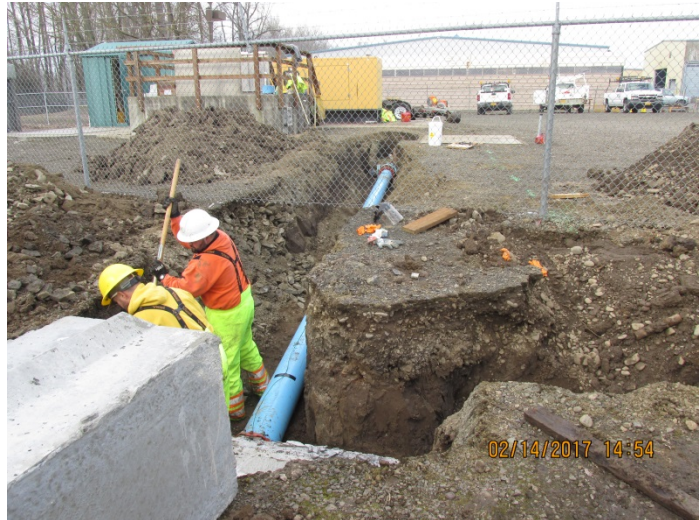
Sewer Repair Project - 2017
