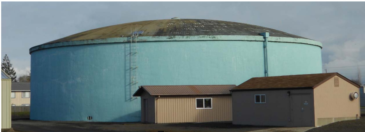
City's 2-Million Gallon Water Storage Tank
