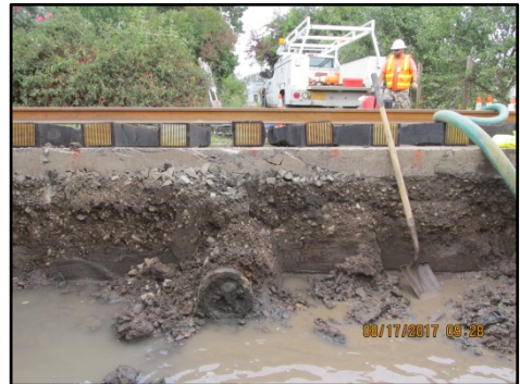
4th Street Railroad Project
