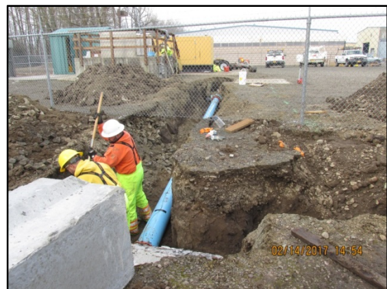
City crews repairing sanitary sewer system
