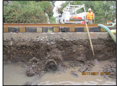
4th Street Railroad Project
