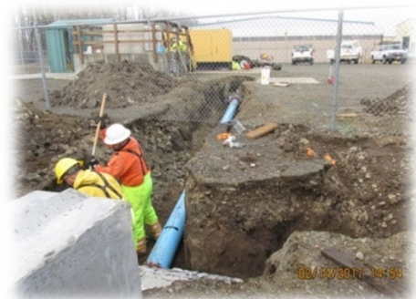
City crew repairing sewer system
