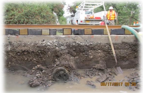
4th Street Railroad Project
