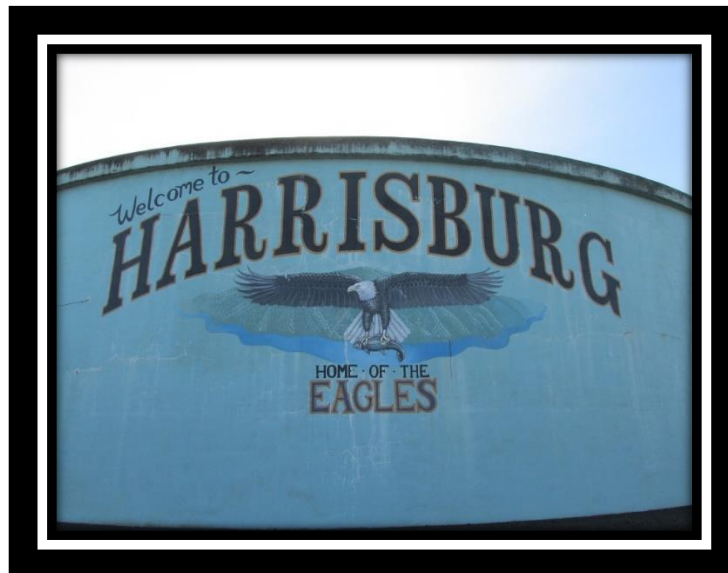
2 M Gallon Water Tank
