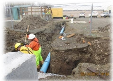
City crew repairing sewer system
