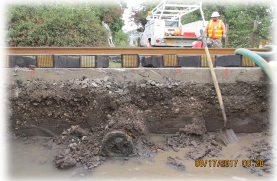
Figure 1 Water Line Replacement
