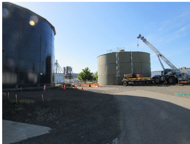
South Water Reservoir Under Construction
