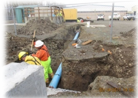
City crew repairing sewer system
