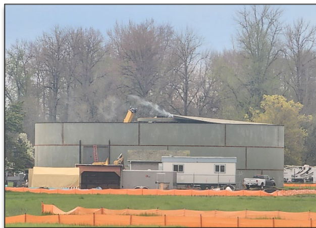
North Water Reservoir Under Construction
