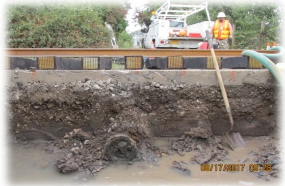
Figure 1 Water Line Replacement
