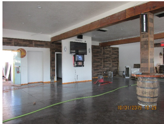
Figure 10: Interior view, (under construction) concrete work & patio entrance
