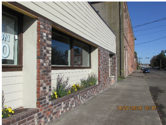
Figure 9: After-View from the corner of Moore & 2nd
