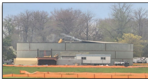
North Water Reservoir Under Construction 1
