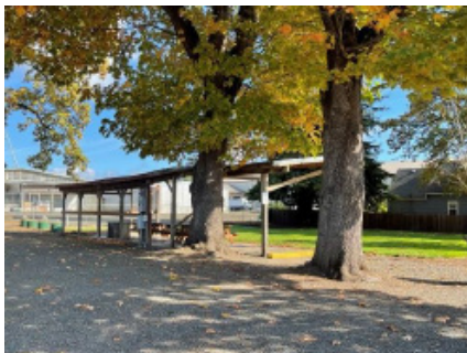
Image 1: View of shade structure and existing tree canopy.
